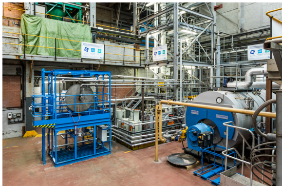
Carbon Clean's skid-mounted, modular carbon capture technology, CycloneCC, shown adjacent to a conventional carbon capture unit at Doosan Babcock's Emissions Reduction Test Facility in Renfrew, Scotland.
